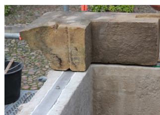
Detail Montage Kranzgesims
